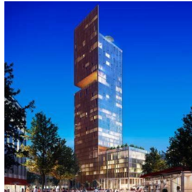
Manhattan Loft Gardens in Stratford MANHATTAN LOFT CORPORATION
