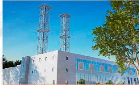
A101 BOILER HOUSE
