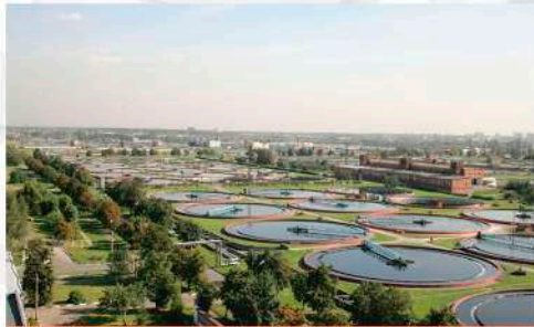
RECONSTRUCTION OF YUZHNO-BUTOVSKIYE SEWAGE FACILITIES
