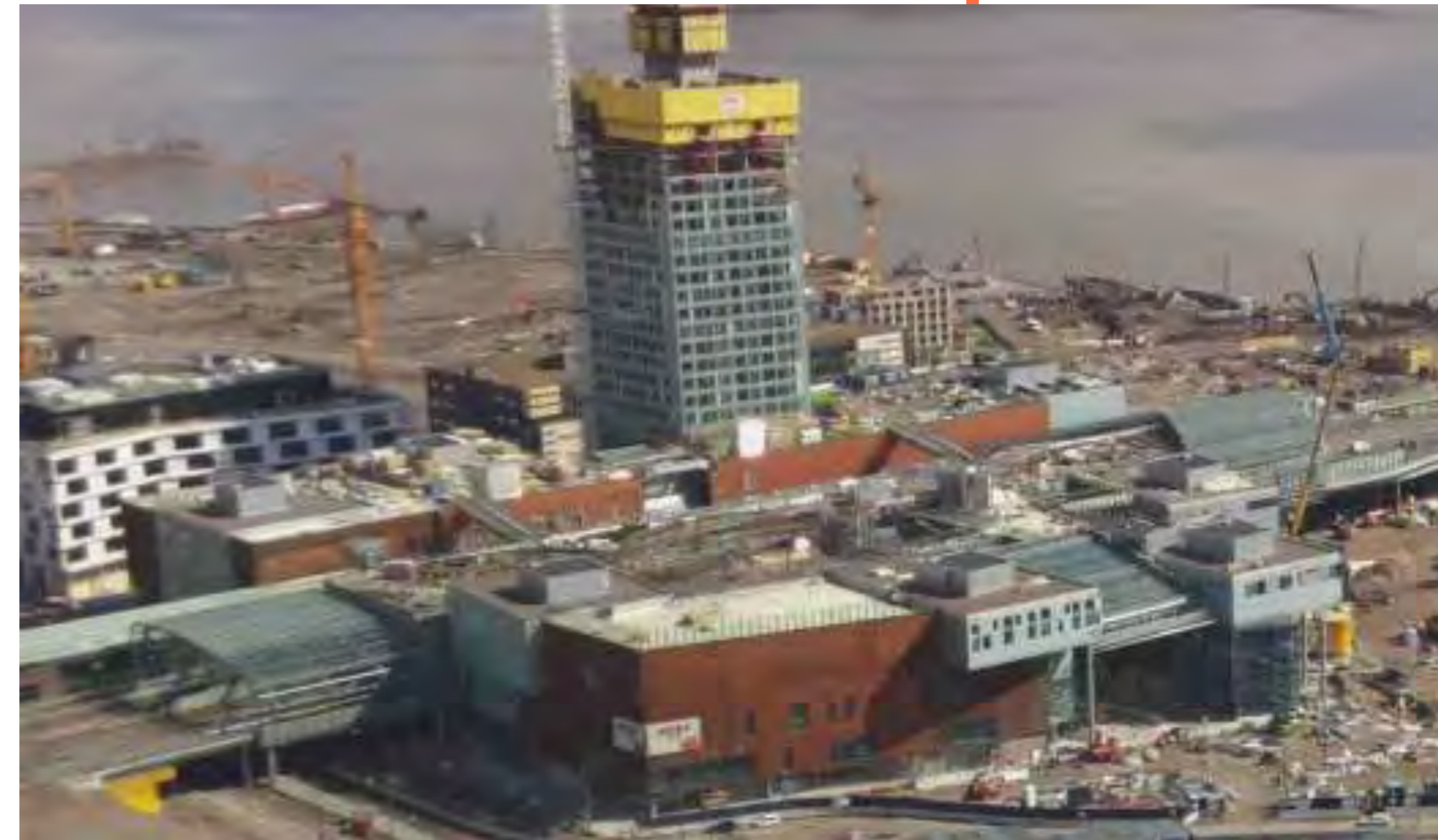
Construction site in April 2018
