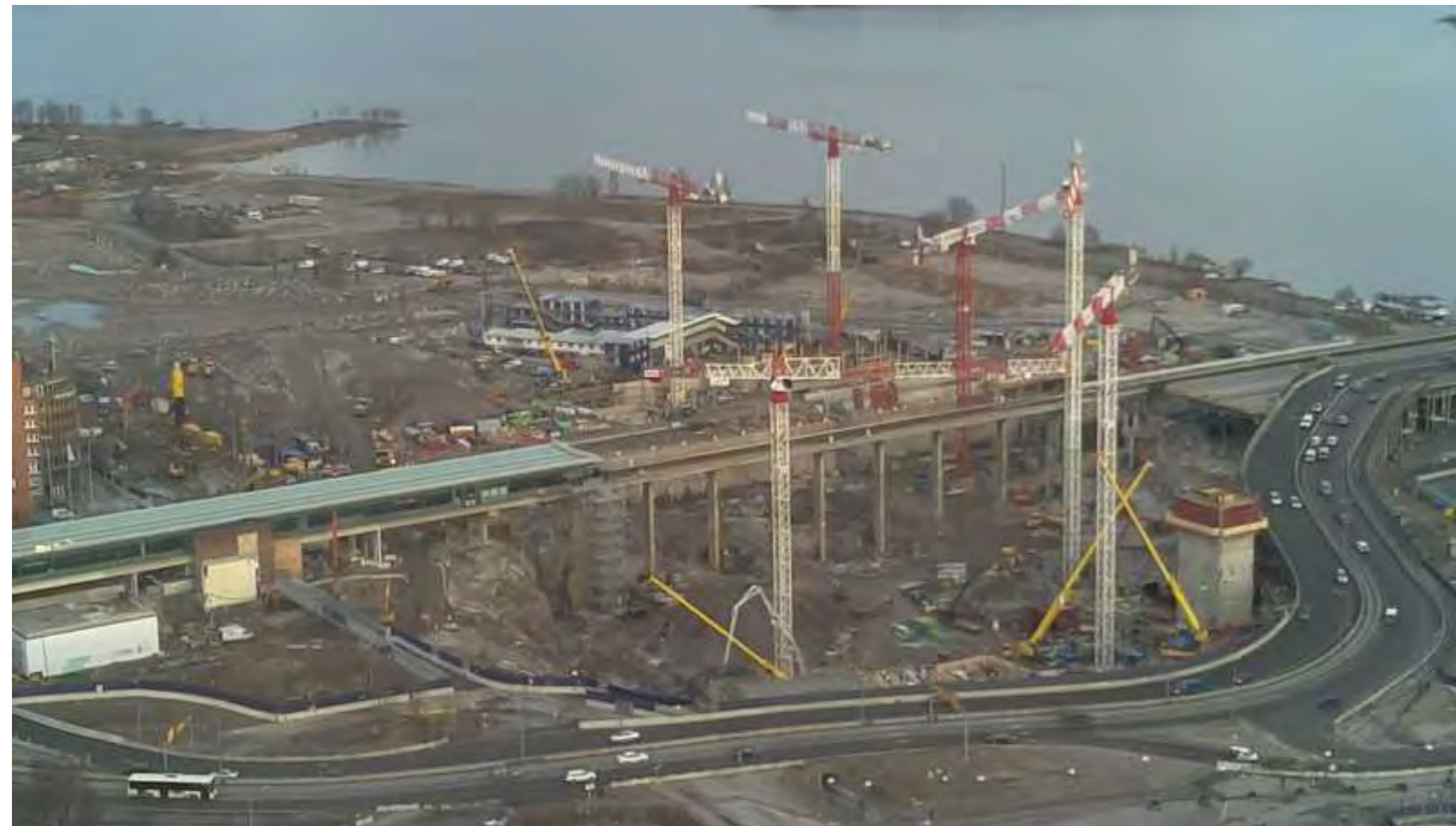
Construction site in December 2015
