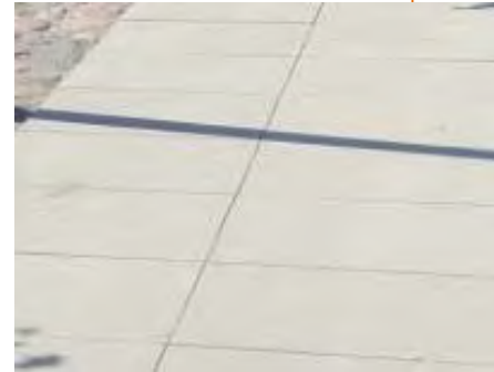
Light concrete pavement
