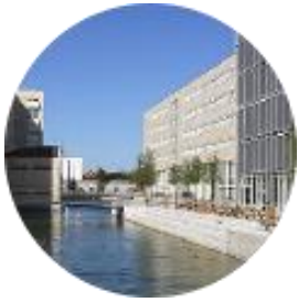
Innovative Rainwater Collection System
